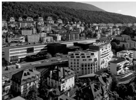
Figure 2: These new buildings, which are easily accessible by public transport, host apartments and professional schools. They were designed to reduce energy consumption.
