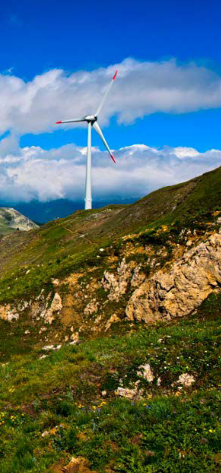
Water dam Griessee and the highest-located wind park in Europe, in the Nufenen region
