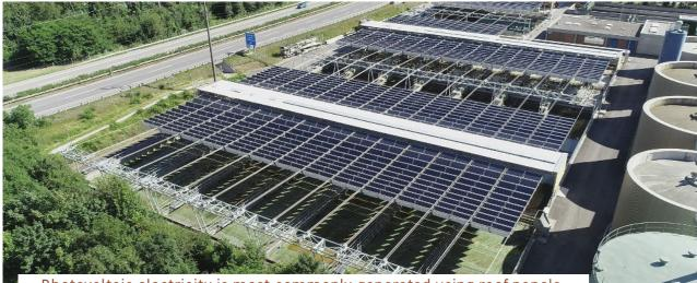
Photovoltaic electricity is most commonly generated using roof panels. But there is considerable additional potential for using other constructions that up to now has been seldom exploited. The solar fold-out roof from dhp technology (in Zizers, Canton of Graubünden) is deployed over treatment tanks in sewage plants to generate renewable energy.
