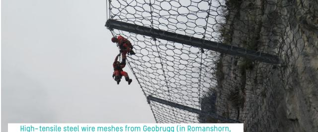
Canton of Thurgau) have been proving their worth for decades as a protective measure against rockfalls, landslides and other natural hazards. In future, the company's products could also help mitigate the effects of climate change.
