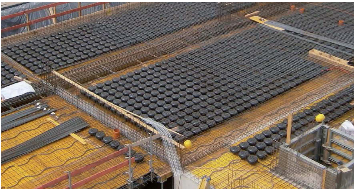
The hollow paving stones from Cobiax
