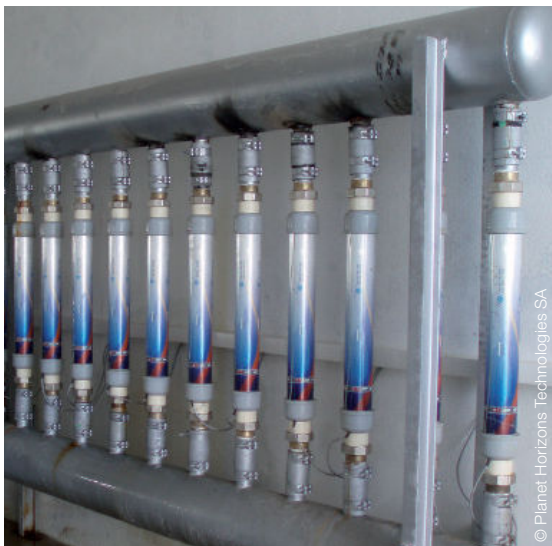
The largest installation provided by Planet Horizons Technologies to date is in Tunisia. The Aqua-4D system treats a throughput of 520 m 3 per hour over an area of 280 ha.
