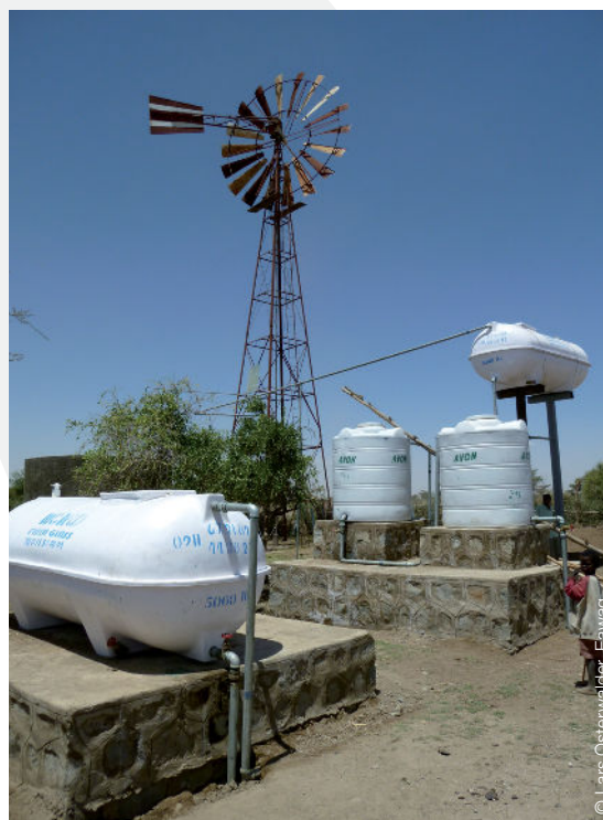
Defluoridation community filter using aluminium hydroxide as filter media, in Tuchi Gragona, Oromia Region, Ethiopia.
