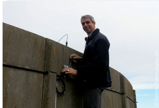
Installed by Cédric Morel, Managing Director of Sensile Technologies, this remote measuring system transmits an alarm if there is an abnormal drop in the level of the slurry pit, thus preventing the pollution of water courses.
