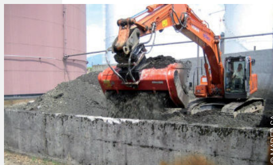
Once blended with soils contaminated with hydrocarbons, these bacteria will digest the pollutants while multiplying until the contaminated site is fully regenerated.
