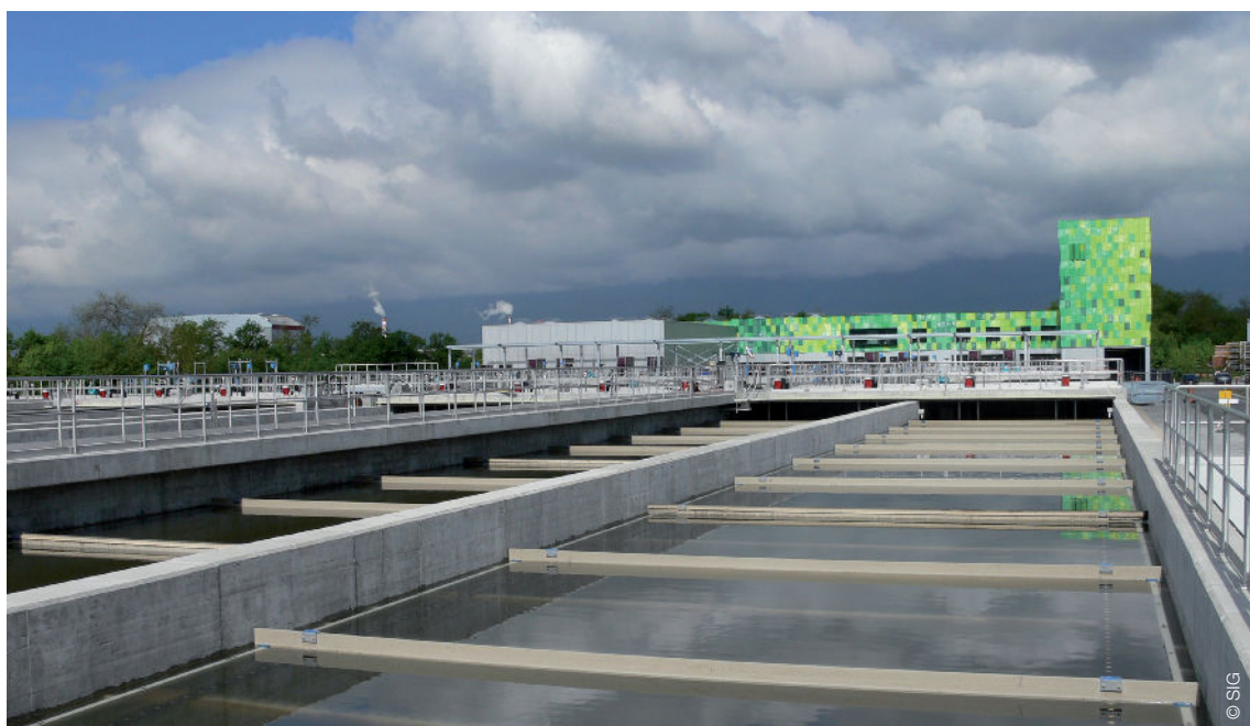
Sewage water treatment plant 'Bois-de-Bay' in Geneva.
